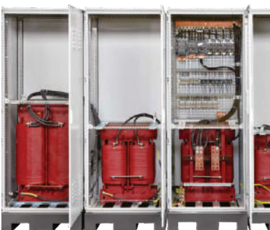
■ Test System for invertors
